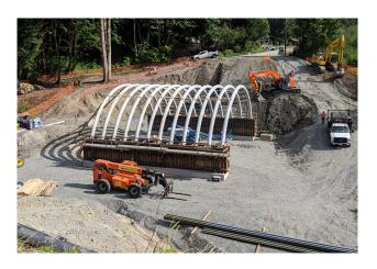
The Composite Arch Bridge System is designed for short span bridges up to 80'.
