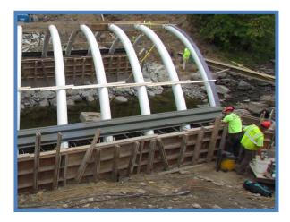
1 x 3 Wooden spacers can be used to maintain the specified arch spacing prior to and during FRP deck installation. AT THIS POINT all arches should be checked and adjusted for plumbness, horizontal and vertical alignment to be within ¼" in each orientation of its intended position.
