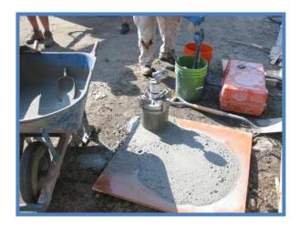
Flowability of the SCC mix is field tested by measuring slump flow. Typically slump flow (measured as diameter of the concrete spread) is between 24"and 30".
