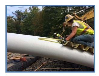
The panels are then attached to the arches using provided fasteners along the spine of the arch. A battery drill with clutch is ideal as care should be taken not to strip holes when fastening the deck. Decking can be field cut to dimensions indicated on the contract drawings. Bevell cutting should be layed out with appropriate project control to assure coordination with embakment slope requirements. Please see AIT details
