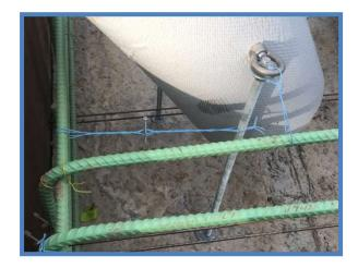
Restraining is accomplished by using AIT provided positioning hardware and fixing the arch end to the abutment at the specified location /elevation. For Bevelled end arch
