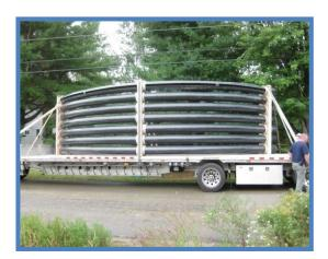
Arches are stacked, crated with blocking as a unit (five to seven stacked arches due to transport height limitations) and shipped on a flatbed trailer from the fabricator. The crate can be unloaded, using an excavator or forklift. The full crate can be offloaded as a
