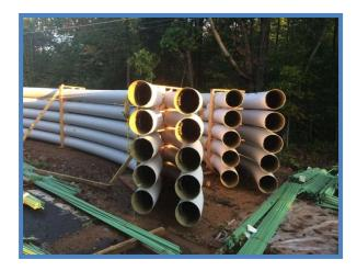
Disassembling arches from the crate is done by hand. Relocating arches to store or set in place by excavator requires one nylon 3" wide sling straps.
