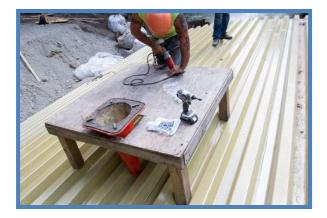
After the arch concrete placement, no other work activities are allowed for 24 hours. Only light foot traffic is allowed over the decking until the arches have reached their desired compressive strength.
