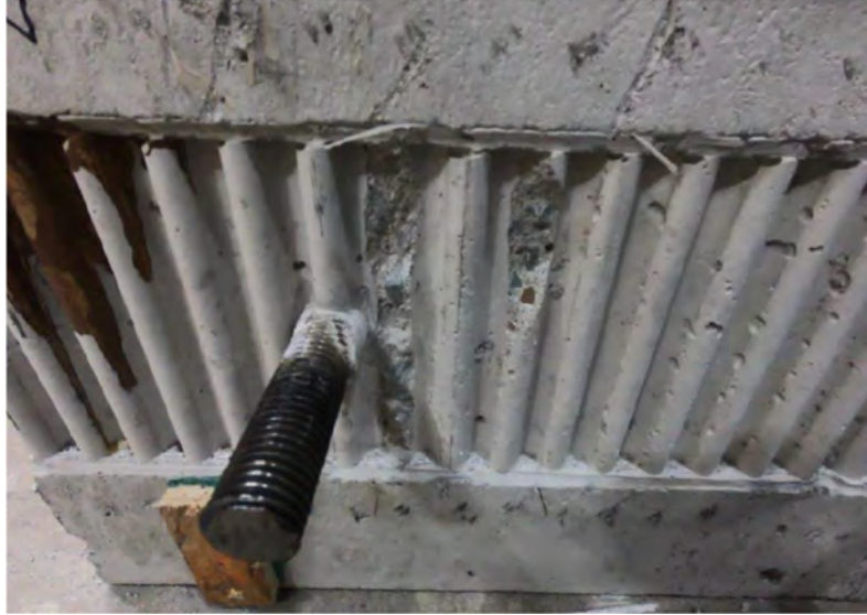
Figure 18: Corresponding Concrete Roughened Surface
