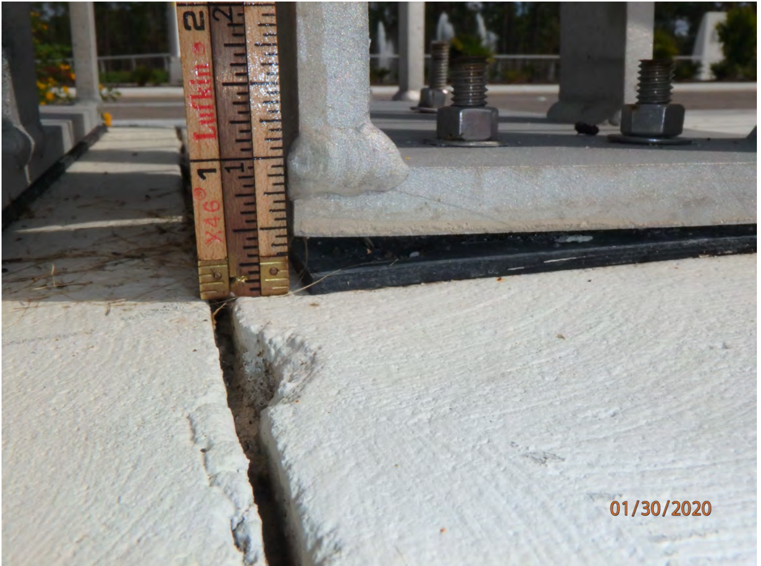
Photo 1 - Element 333/3 Other Bridge Railing
