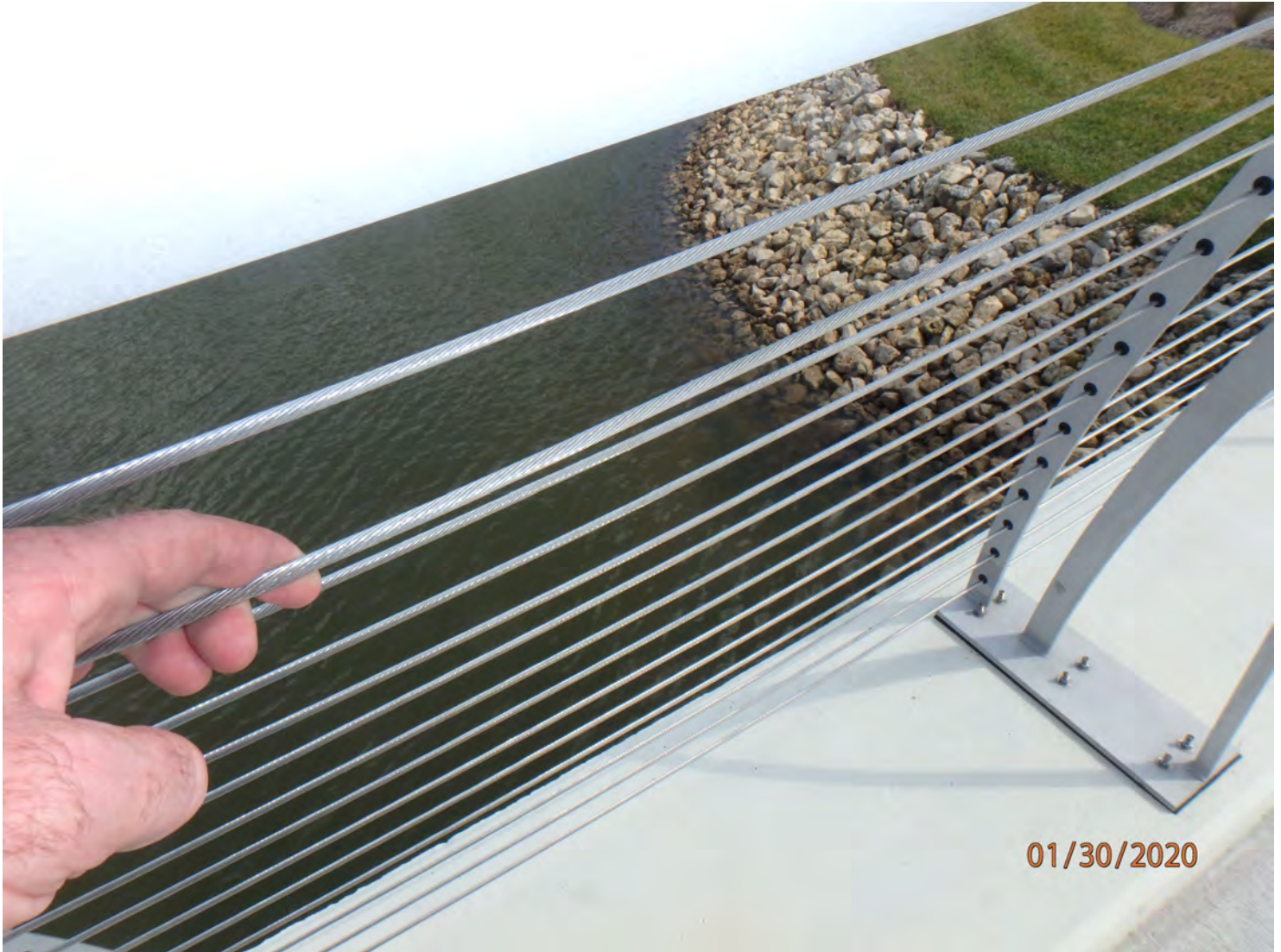
Photo 2 - Element 333/3 Other Bridge Railing
