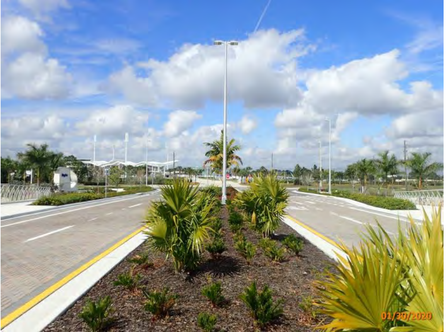
NORTH APPROACH LOOKING NORTH
