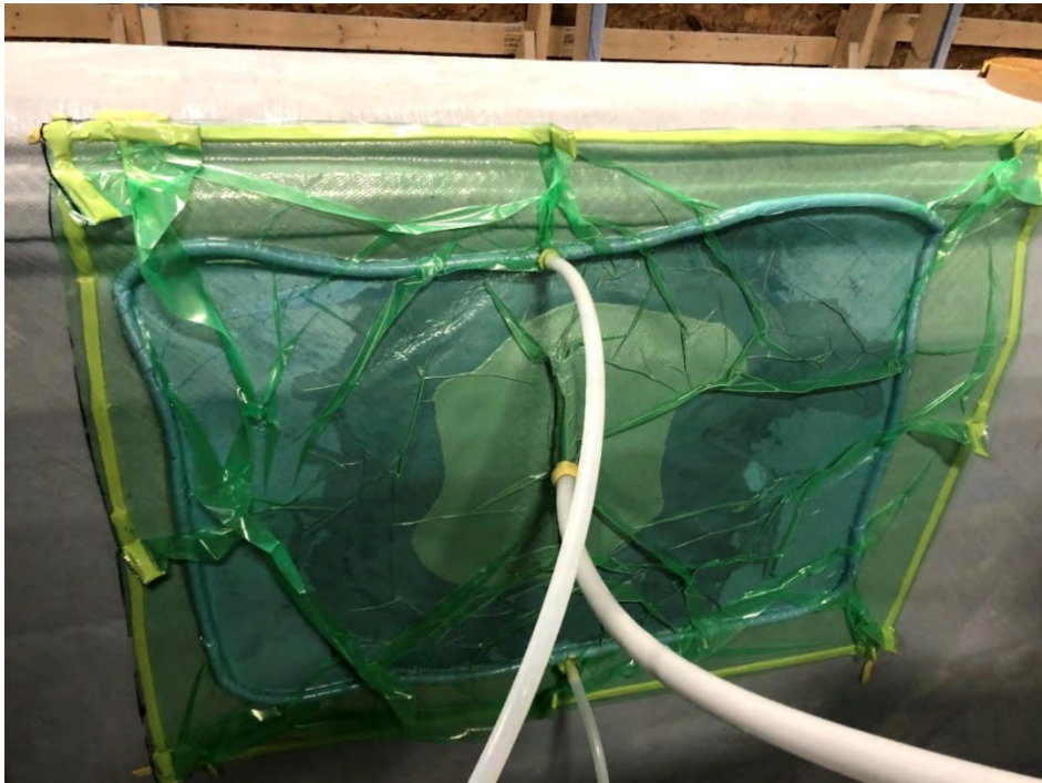
Figure 33: Repair Infusion
