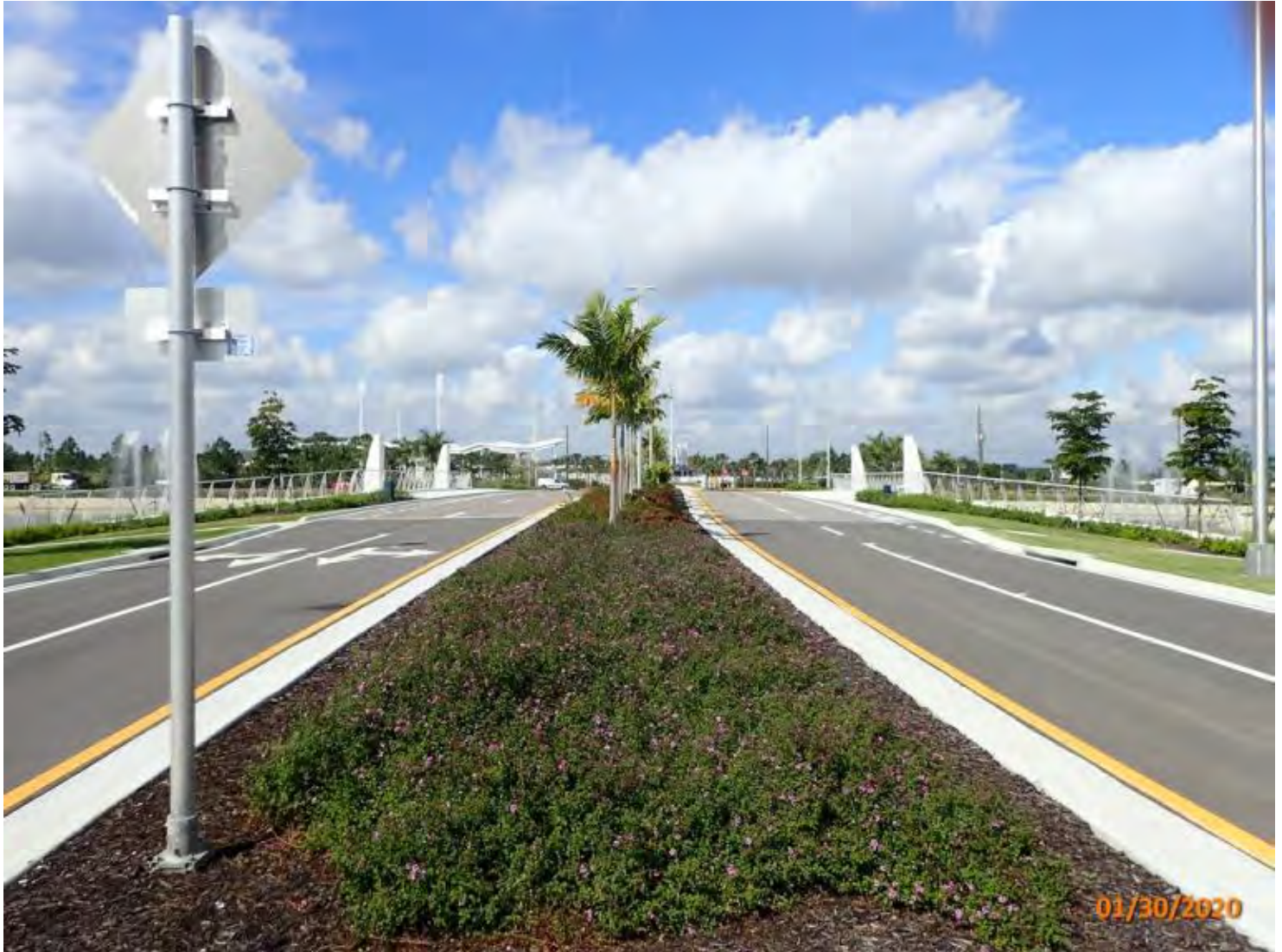
SOUTH APPROACH LOOKING NORTH
