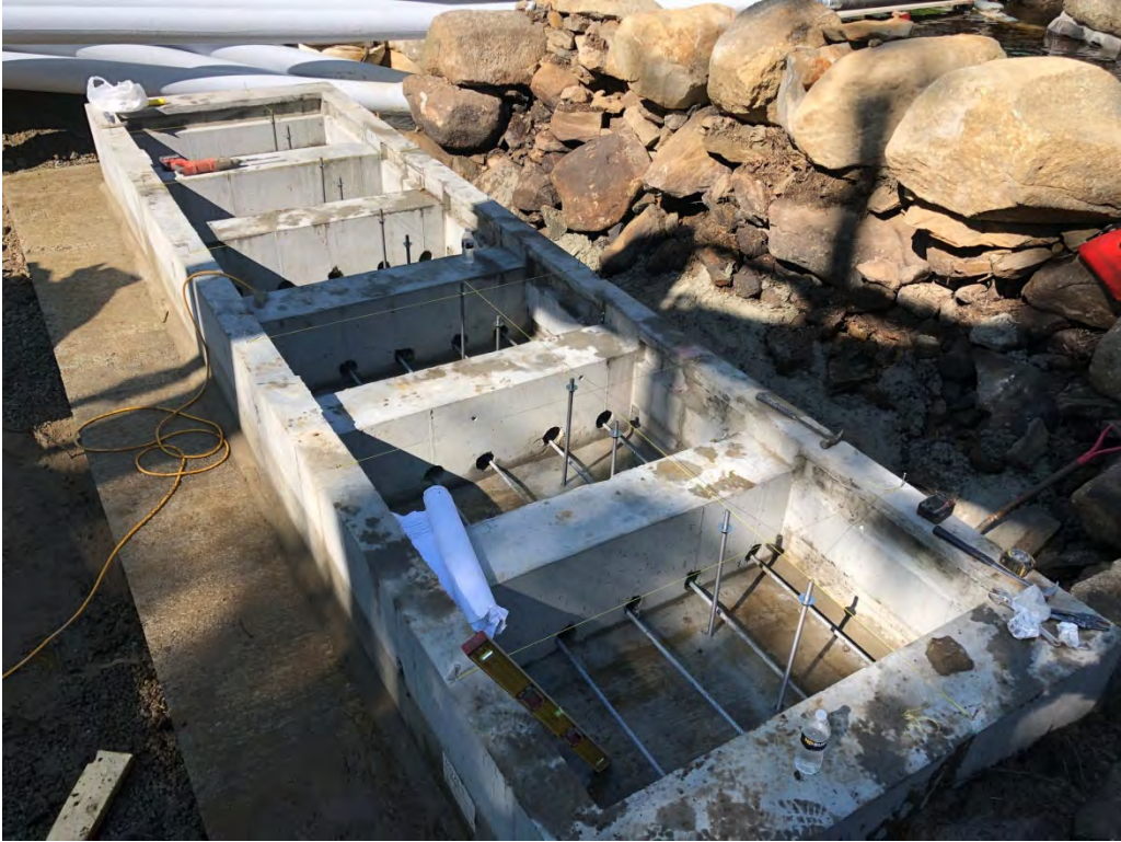
Figure 8 Precast Concrete Foundation for GArch System
