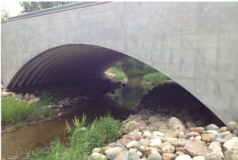
Figure 14: Precast Cantilevered Headwall
