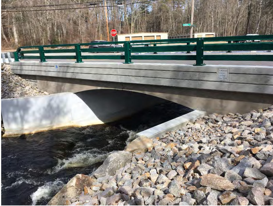
Figure 11: Precast Through-Tied Headwall
