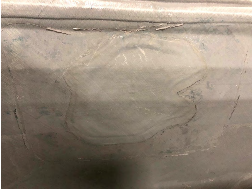
Figure 34: Completed Major Repair
