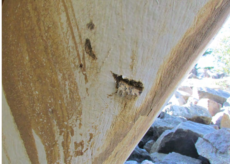
Figure 24: Example of Laminate Gouging
