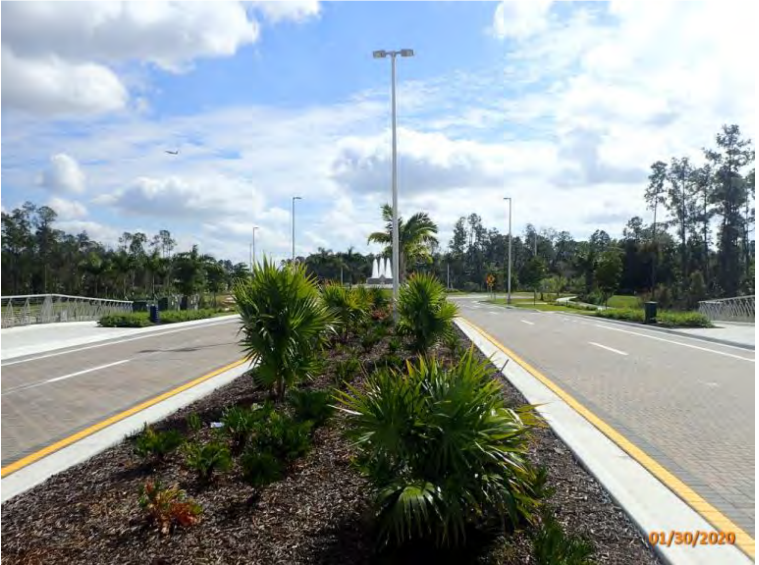
SOUTH APPROACH LOOKING SOUTH
