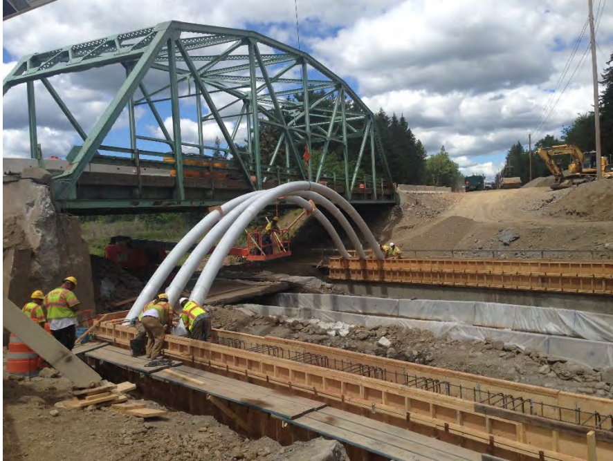
Figure 10 Cast-in-Place Concrete Foundation for GArch System
