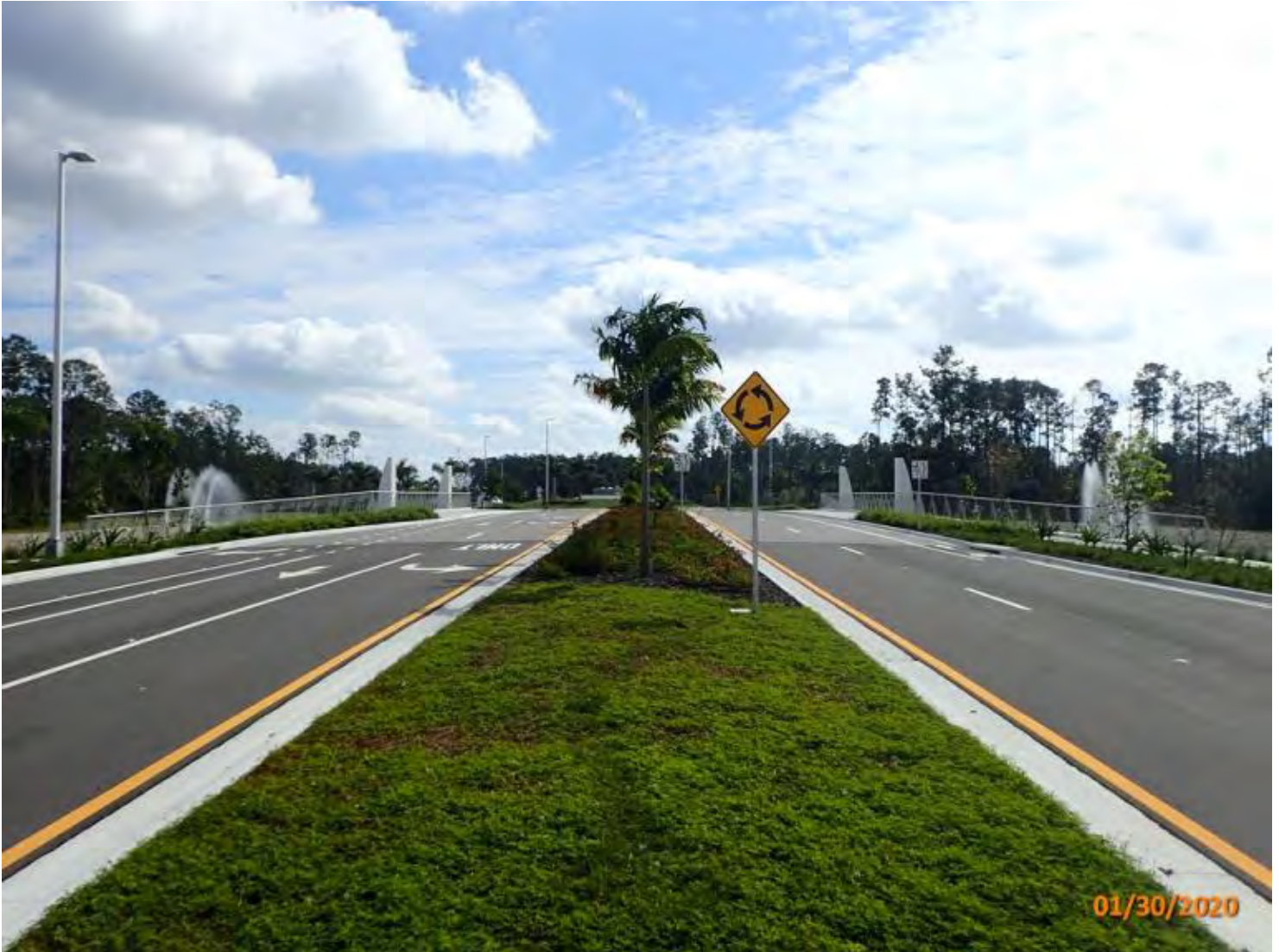
NORTH APPROACH LOOKING SOUTH
